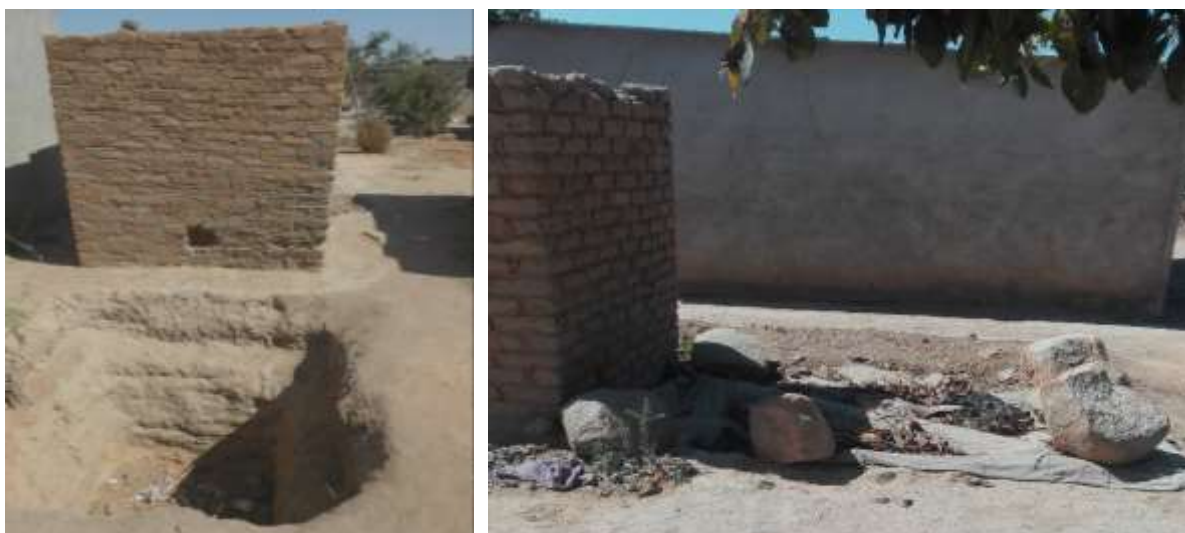
Figure 8 Left: Toilet under construction with a hole in the ground to contain the excreta;
