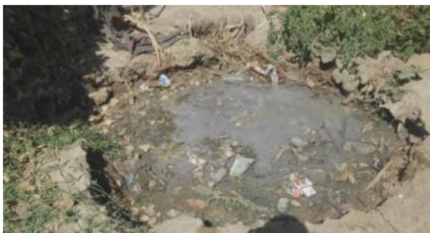
Figure 9 A sewage pit filled with faecal matter exposed to the surface
