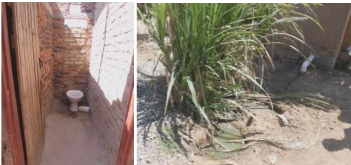
Figure 7 Left: Sanitation facility with only a seat and no water tank for flushing; Right: Raw sewage flowing to the outside
